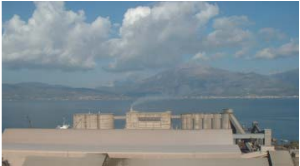
Fig. 1: Continuous emission monitoring is a matter of growing concern
